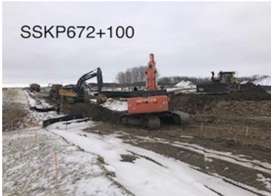
Water Course Unnamed drainage SK WC74 SSKP672.1 Excavation
