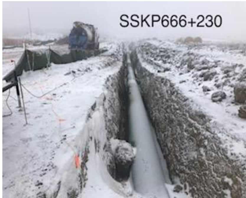
Hydro Vac truck de-icing and draining mainline section before backfill
