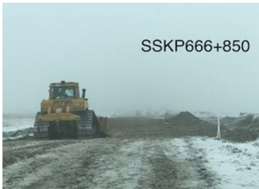
D6 levelling the right of way making accessible for pipeline equipment and trucks
