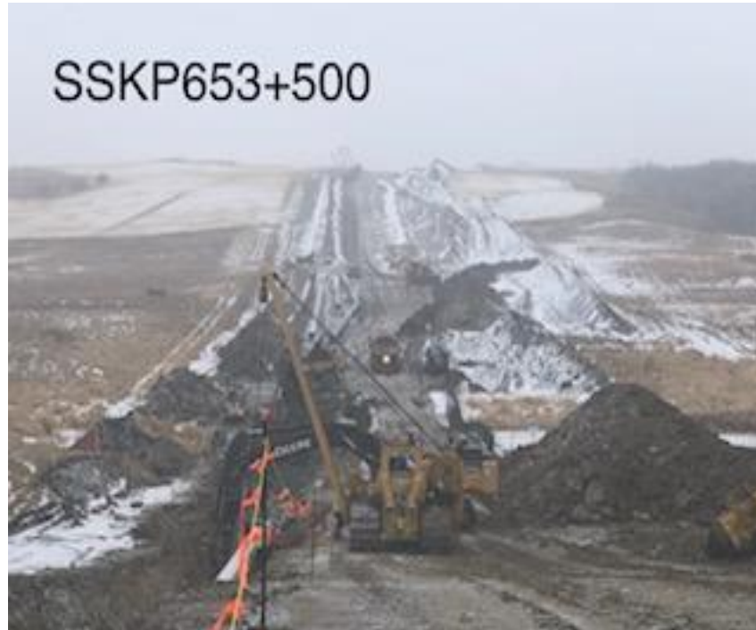
Water Course Vipond Creek SK WC72 SSKP653.52 Excavation
