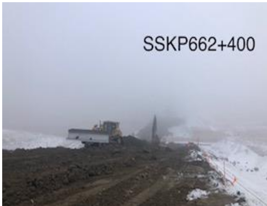
Backfill continues at Vipond creek SK WC72
