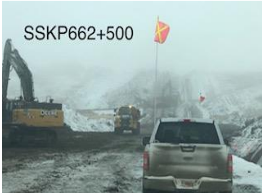
Backfill at Vipond Creek SK WC72
